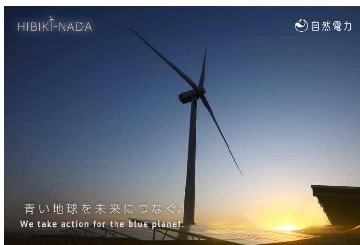
Kitakyushu Hibikinada Wind & Solar Power Plant (Introduction movie: https://youtu.be/YJdg365cDBw )
