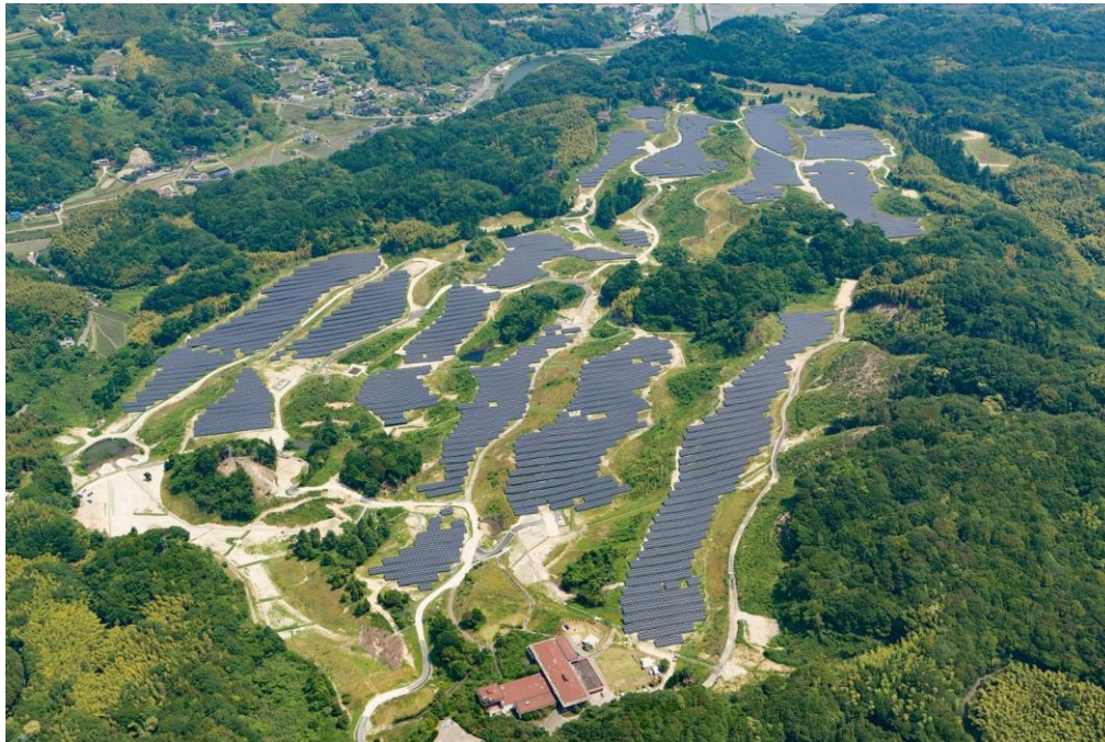
Panoramic view of the power plant
