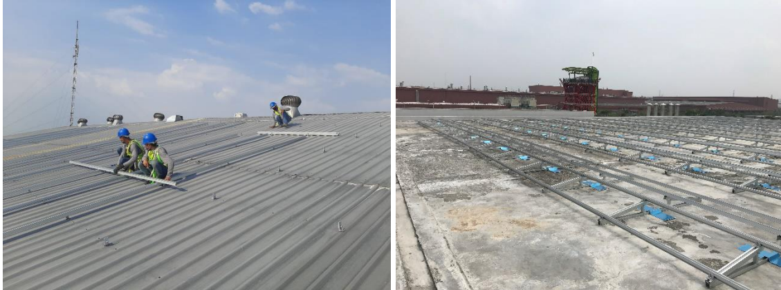
[Pictures from the construction sites]
