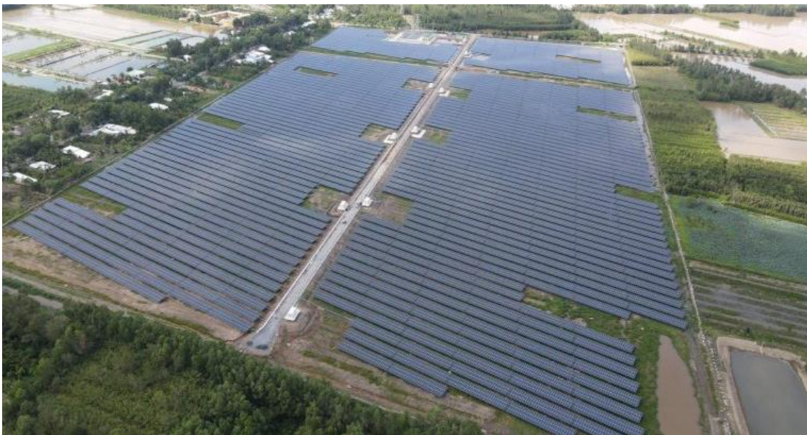
Hau Giang Solar Power Plant
