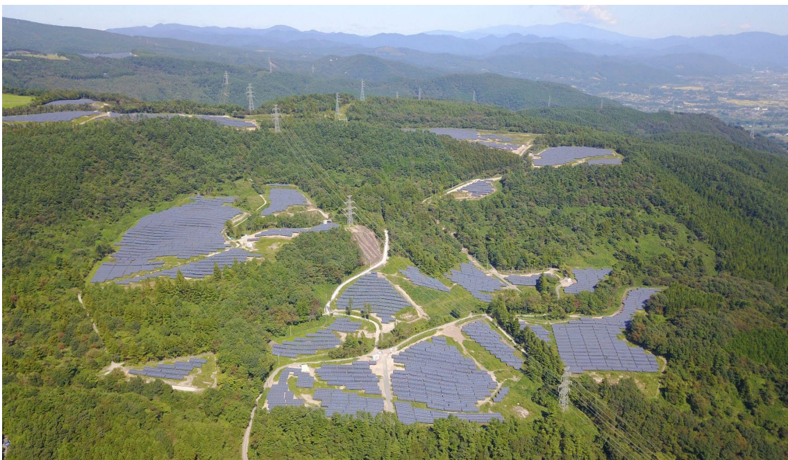
*The photo shows the part of this power plant.
